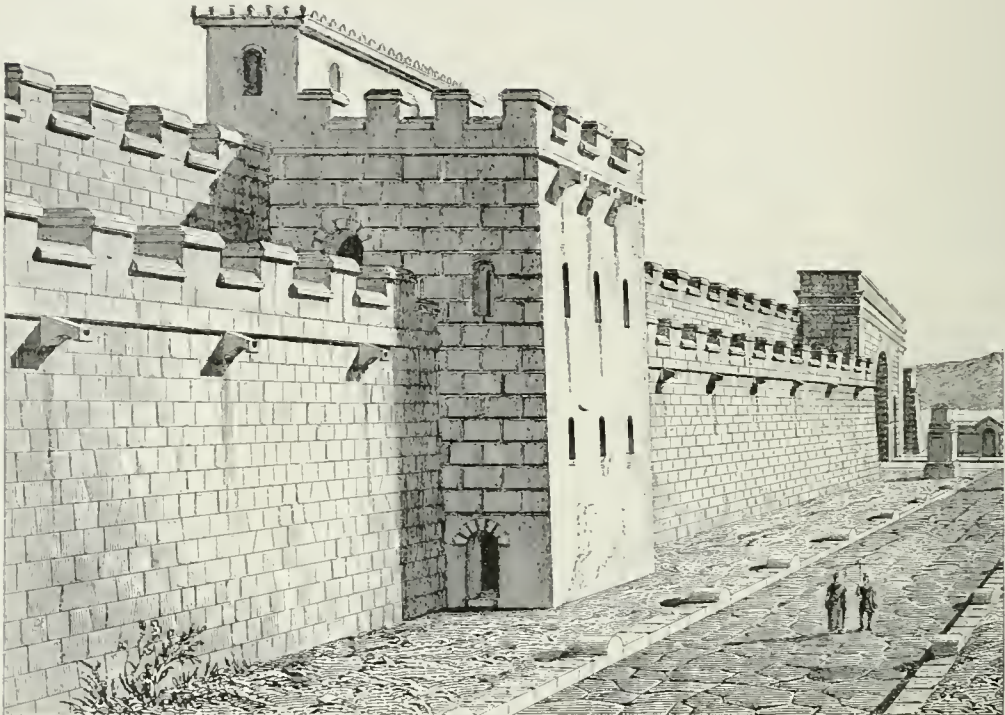
RAMPART CARRYING AN INNER AND AN OUTER CRENELATED PARAPET, ALLOWING OF TWO LINES OF BOWMEN, ETC. WALLS OF POMPEII, CAMPANIA, ITALY; PROBABLY C. 200 B.C.
